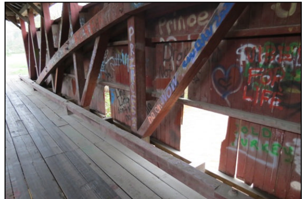
Photo at left shows damage to Keefer Station Bridge likely from vandals and probably some storm damage at bottom boards. Photo at right shows graffiti in Keefer Station Bridge.
