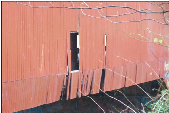
Photo at left shows damage to Keefer Station Bridge likely from vandals and probably some storm damage at bottom boards. Photo at right shows graffiti in Keefer Station Bridge.
