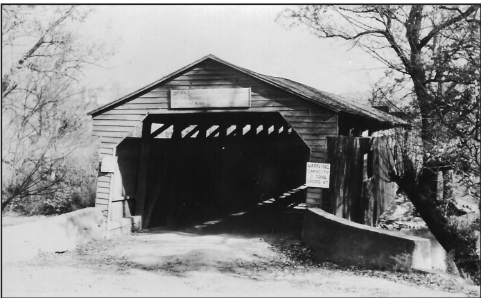
Shermansdale Bridge crossed Sherman's Creek, west of SR 74 at Shermansdale in Carroll Township, Perry County. The bridge was a one span, Burr Arch truss, 174 ft. in length. It is not known when it was built but it collapsed in 1945.
