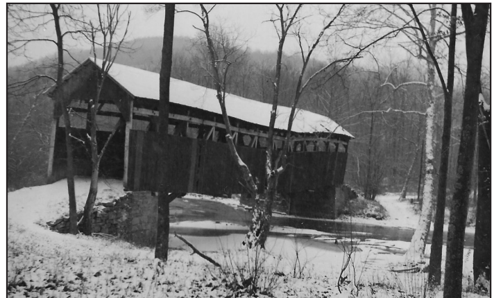
Upper Humbert Bridge, PA-56-04, shown photographed here on December 10, 1961, spanned Laurel Hill Creek. Built in 1891, it was located northeast of Ursina in Lower Turkeyfoot Township. The 120 ft. Burr Arch span was burned in 1969.
