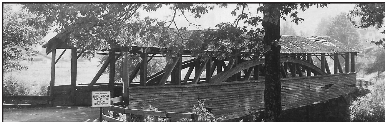
Watrous Bridge crossed the west Branch of Pine Creek at Watrous off Rt. 6, east of Galeton, PA in Tioga County. Built in 1859, the 100 ft. Burr Arch truss span was replaced in 1937.
