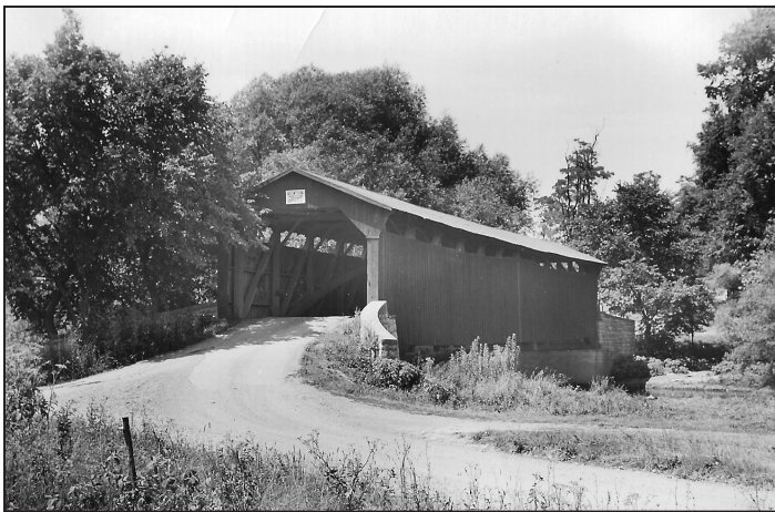
Naugle Bridge spanned Buffalo Creek with a 150 ft., Burr Arch truss. It was built in 1876 by Peter Kiefer of Sunbury, PA, who was credited with building many covered bridges in Union and Snyder Counties. It was located northwest of Lewisburg, PA in Union County in the area known as Dale's Ridge. Unfortunately, it was torn down in 1955.
