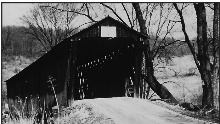
Hoover or Toad Hollow Bridge, PA-32-02, was located on LR 32177 South of Smicksburg in West Mahoning Township, Indiana County. The bridge was a Town Lattice truss 112 ft. in length across Little Mahoning Creek. Built in 1881, it was replaced in 1960. This photograph was taken by Thomas Sutter in March 1959.
