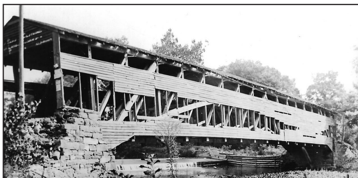
Price Bridge crossed Muncy Creek at Shady Nook Park near Hughesville in Lycoming County. The bridge was located near the junction of SR 405 and US 220. The missing sideboards reveals that it was of Burr Arch truss construction.
