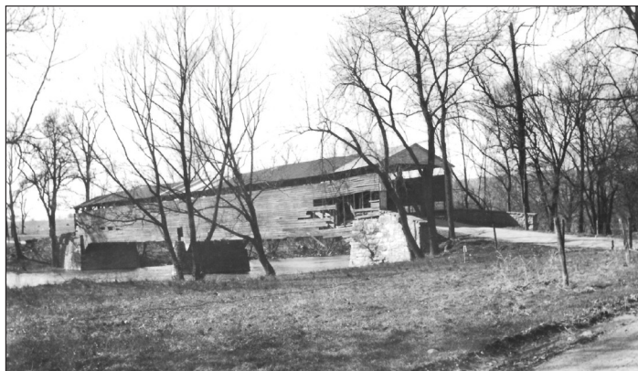
Bernheisel Bridge was also known as Hoover's Bridge. It was a 2-span, 195 ft. Burr Arch truss span across Conodoguinet Creek. It was located in Middlesex Township, Cumberland County, on present day Bernheisel Bridge Road, T-574. It was built in 1869 by John Gutshall for $2885.59. It replaced an 1843 bridge built on the same site. The above shown bridge was replaced in 1959 by a steel and concrete bridge.
