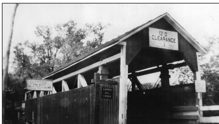
Trent Bridge spanned Laurel Hill Creak on LR 54049, Copper Kettle Highway, in Middle Creek Township, Somerset County. It had a 12 ft. 0 inches clearance height and was about 80 ft. in length. The Burr truss span was replaced in the late 1950's or early 1960's.
