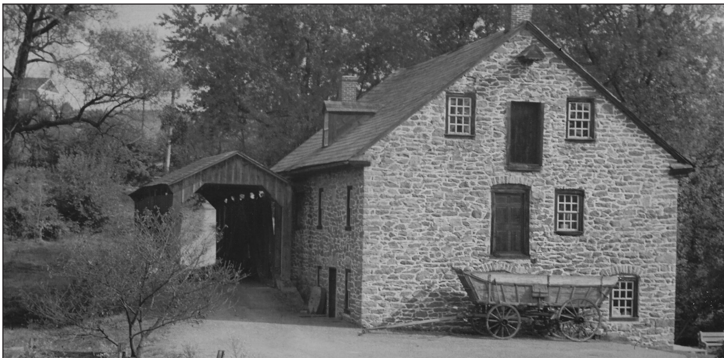
John Stoner's Mill or Jacob Mann's Mill Bridge, PA-36-17, was one of those increasingly rare covered bridge and mill combinations. The three-story stone gristmill was built in 1779 and the covered bridge was built much later in 1868 by renowned Lancaster County covered bridge builder, Elias McMellen. The bridge was a 65 ft. long, Modified Kingpost truss and cost $1700. It spanned Little Conestoga Creek between Lancaster and Manor Townships on School House Road, T-595, Lancaster County. The gristmill was on the Manor Township side of the township boundary line. Unfortunately, the covered bridge was lost during Tropical Storm Agnes on June 22, 1972.
