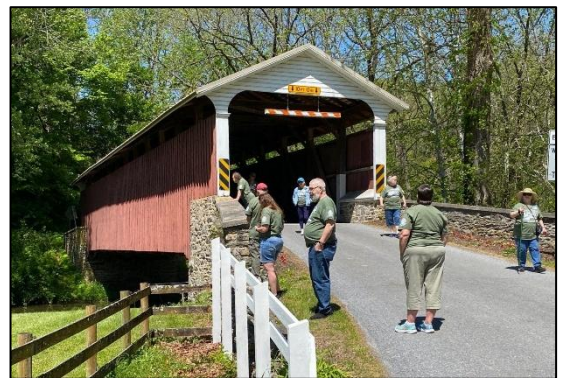
Mercer's Mill Bridge
