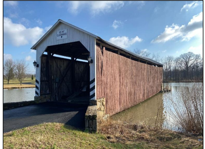
Anderson Farm / Mud Run Bridge Photo by Jim Smedley, March 21, 2026.
