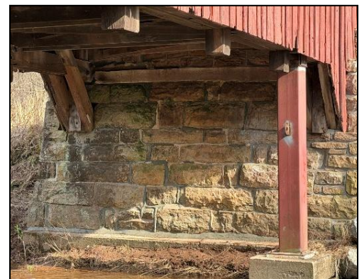
Photo of repaired abutment courtesy of Historical Society of Perry County.
