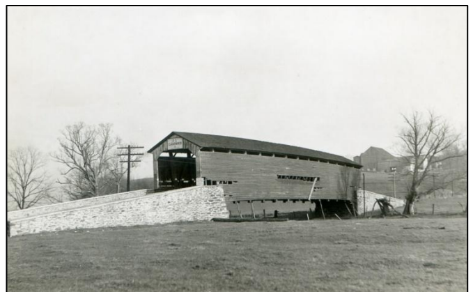
Bellbank Bridge connected Chester and Lancaster counties. This Double Burr arch truss bridge was built in 1861 and lost to arson in 1979. It crossed the East Branch of Octoraro Creek. RPPC postcard, c1950s.
