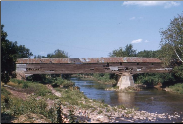
PA-67-01x Detter's Mill Bridge in 1958. Built by John Finley in 1849, this 2-span, 175-foot bridge crossed Conewago Creek. One span collapsed in July 1965. The remaining span was destroyed by arson in 1966.
