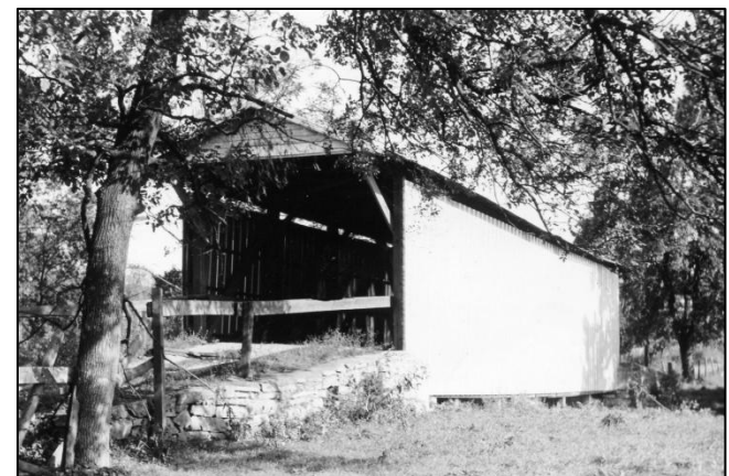
PA-67-33x W. H. Dietz's Farm Bridge crossed Kreutz Creek between Hallam and East Prospect in Hellam Township. This short 72-foot, Burr arch truss bridge was built in 1836 and replaced in 1956.
